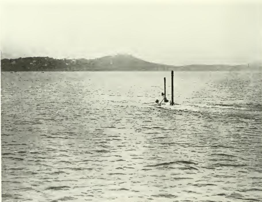
Submarine running submerged, with periscope exposed.
