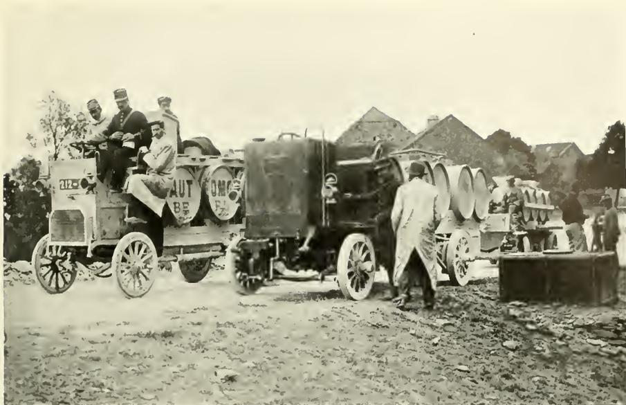
French tank motor-trucks for carrying pure water.
